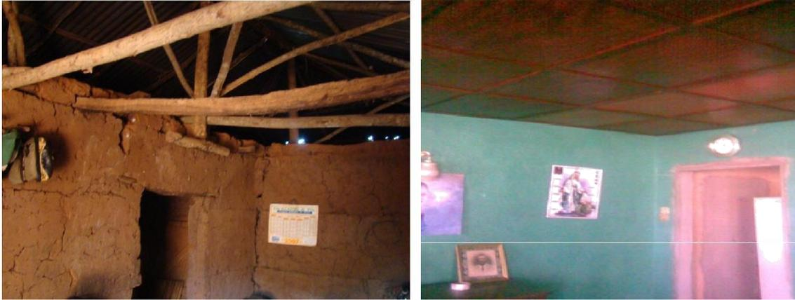
**Figure 5.** A) Habitat showing a lot of space between the rough wall and the roof with several cracks in the wall (Dangbo); B) habitat with a ceiling and smooth wall without cracks or spaces (Dangbo).
